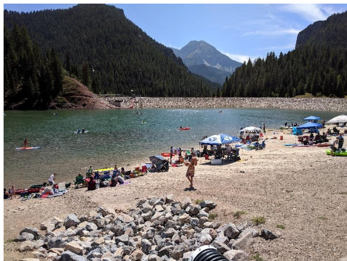
Figure 2. Tibble Fork Reservoir, Utah County.
